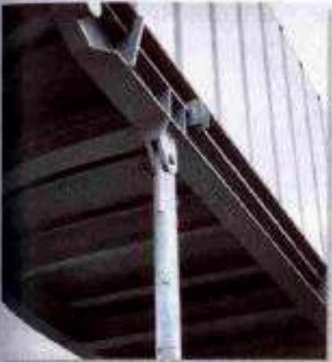
The cable exerts a force on the bracket in the direction of the cable. (1)
