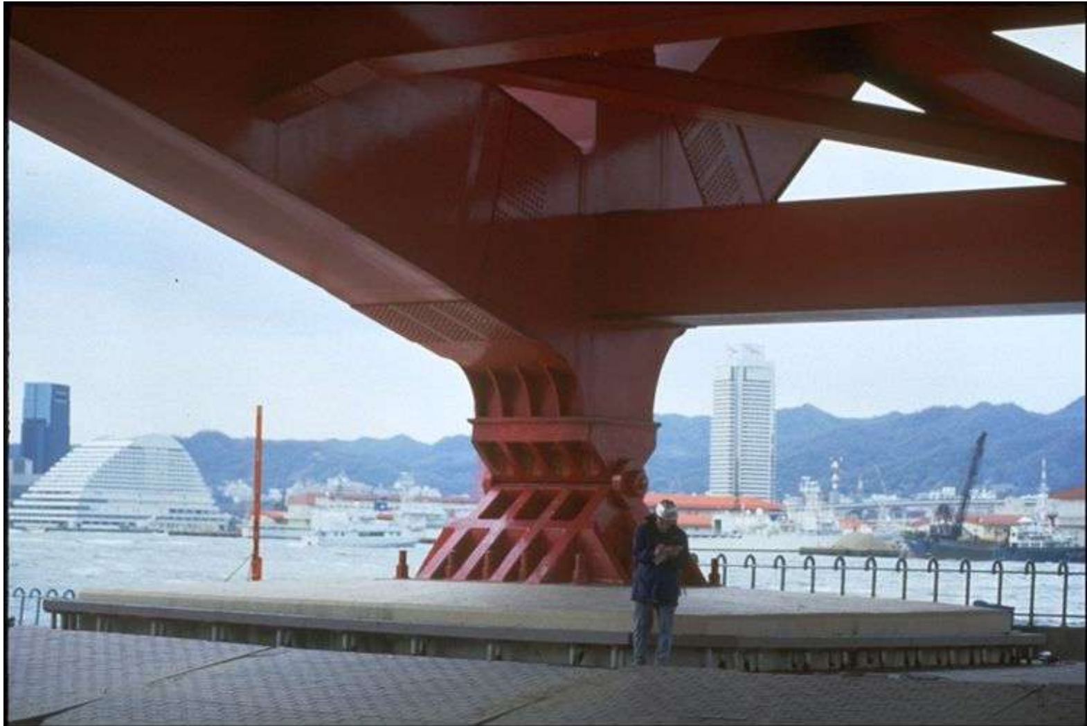
Description: Southside arch support (Port Island Bridge)
